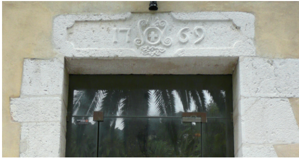
◀ Fig. 13 : Le linteau de la porte principale du bâtiment des galériens (photo J.-C. Braconnot). Lintel of the main door of the galley slaves hospital with the date of the end of its construction.
